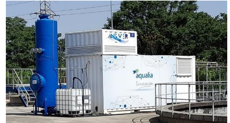
Pilot: electrostimulated anaerobic reactor
