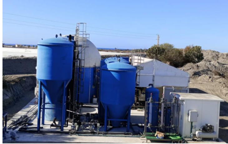
Combined treatment of Urban Waste Water (WW) and the Organic Fraction of Municipal Solid Waste (OFMSW) in WWTPs with positive energy balance for small populations (less than 50,000 IE).
